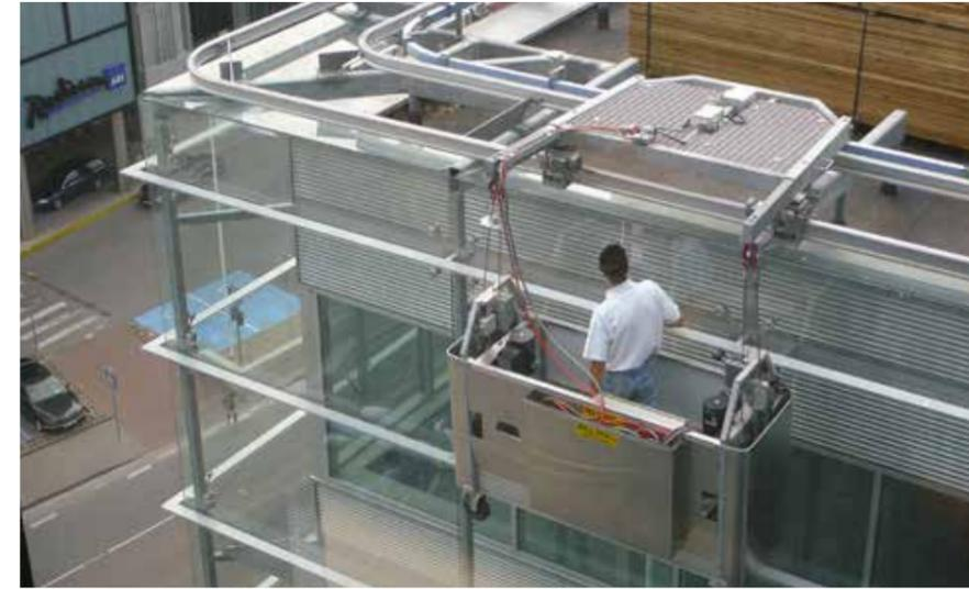
A light roof trolley is an extremely flat machine traversing on two parallel tracks. The roof trolley consists of one or two suspension jibs. The suspension jibs can be either foldable (with fixed outreach from the facade) or telescopic (adjustable outreach). With both suspension alternatives, the jibs are moved out of sight when the roof trolley is not in use.
