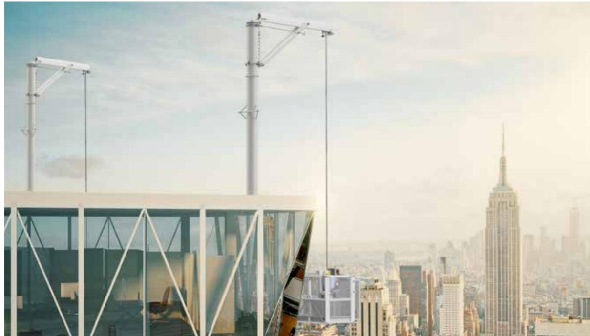
A davit looks like a simple, small crane used for suspending platforms. A davit system consists of two main parts: the portable davit and the base plate or pedestal. The davit is the visual part and the base is plate mounted to the roof to which the davit is attached to.
