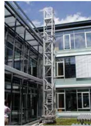
◀ With box ladders it is possible to safely climb inside the ladder. The box ladder can traverse easily with an electrical motor or manually along the tracks mounted on the building.
