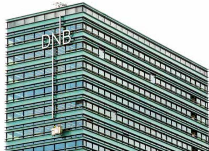
The best thing about our roof trolley system is that it is hidden on top of the roof when not in use. It is almost non-visible from the street below and from neighboring buildings. It doesn't excessively increase the height of the building. Also a roof trolley weighs less than 300 kilos (700 lbs.) and twin aluminium tracks are less than 15 kilos (33lbs) per meter. The Rostek roof trolley system is therefore suitable for even light roof structures.
