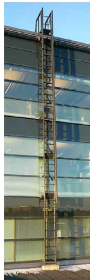
▲ Manual traverse is the normal way of moving a ladder. A ladder can also be driven up and down along an inclined glass roof with electrical motors or with hand crank trolley.
