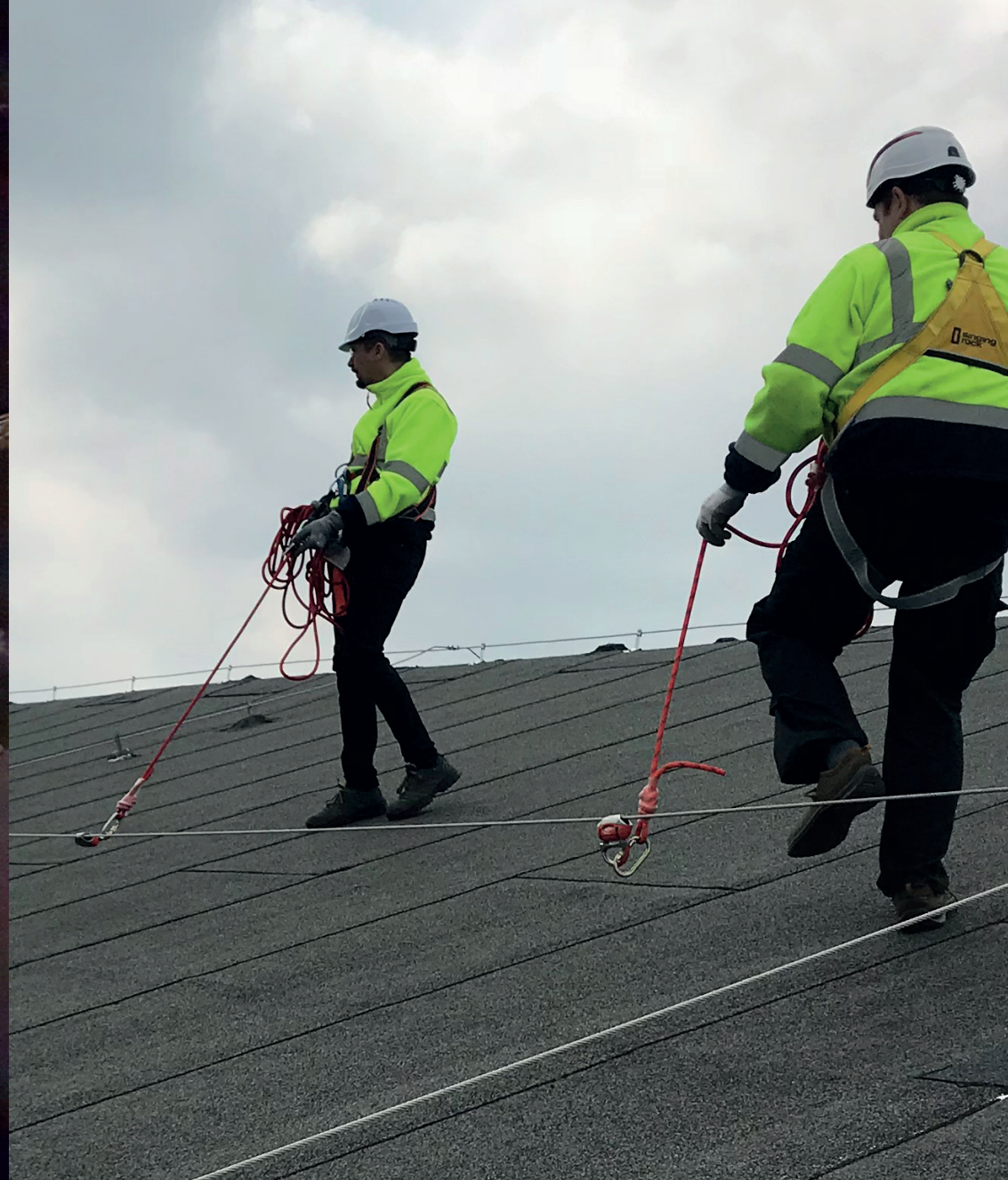
5. Rope system with a guided type fall arrester
