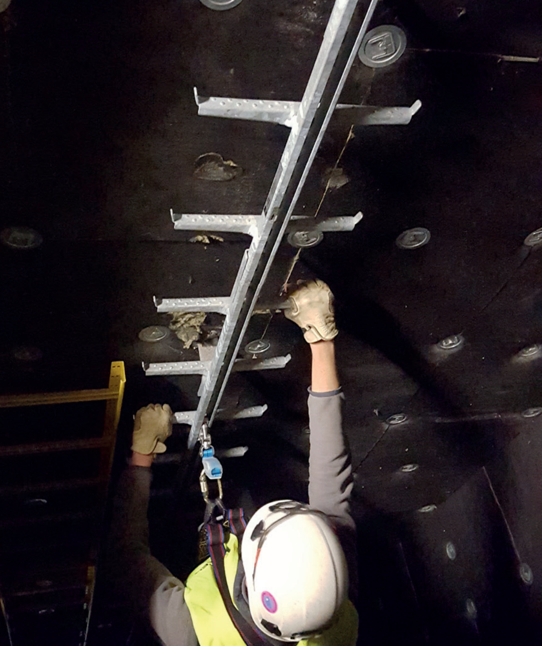
4. Vertical system with a rigid anchor line
